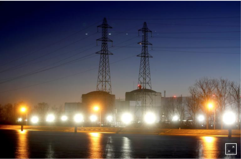
FILE PHOTO: A night view shows France's oldest Electricite de France (EDF) nuclear power plant and the Grand Canal d'Alsace near the eastern French village of Fessenheim, France February 20, 2020. REUTERS/Arnd Wiegmann
